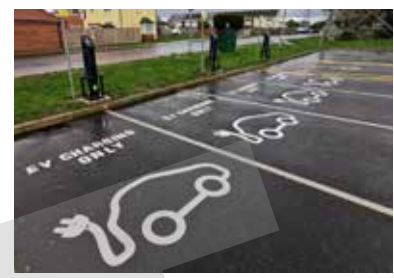
EV Chargers, Lynnsport
